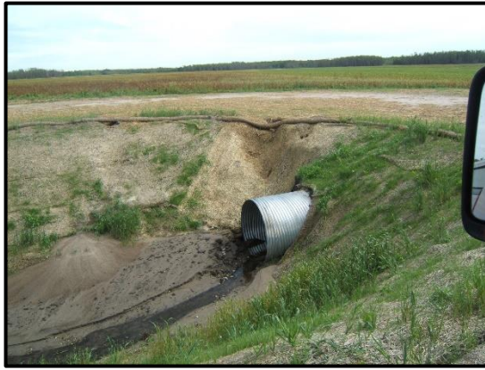
Erosion around access crossing
