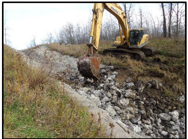
Placing rip-rap in the erosion hole
