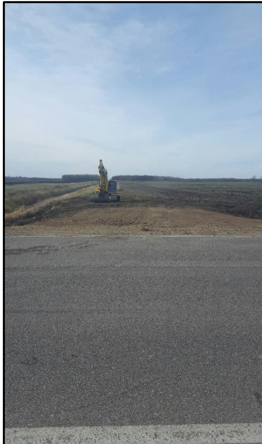
Finished access crossing - 30' top width
