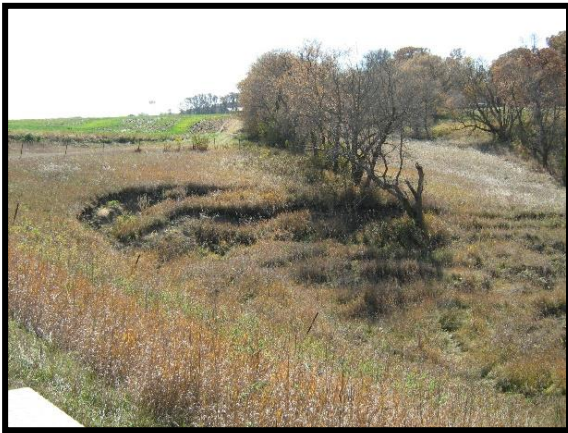
Slope failure/deteriorated metal control structure
