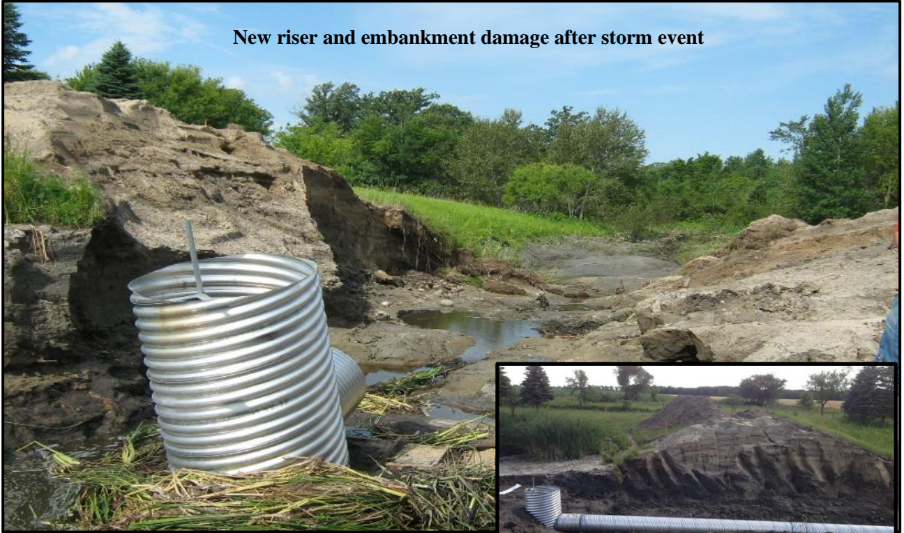
New outlet structure ready to back fill
