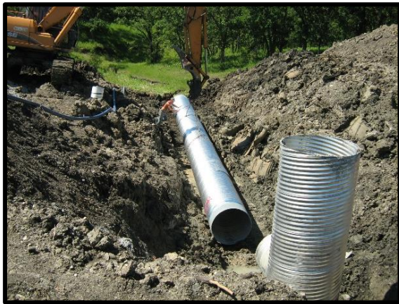
New control structure installation
