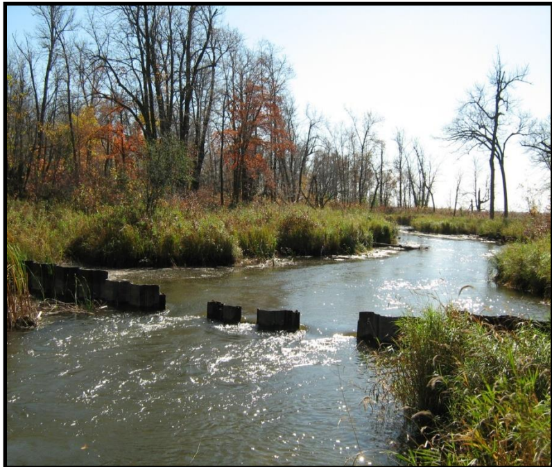
Typical fall drawdown with stop-logs removed
