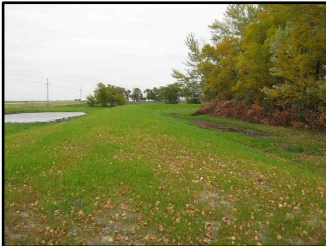
North levee wall
