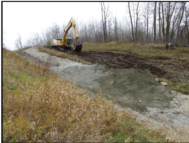
Completed repair of the failed chute
