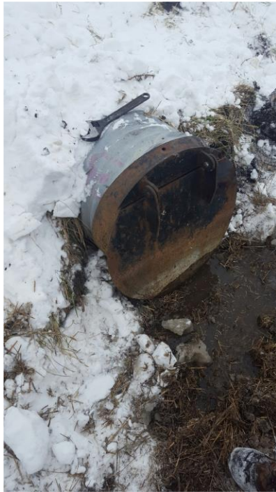
End of pipe and trap repaired
