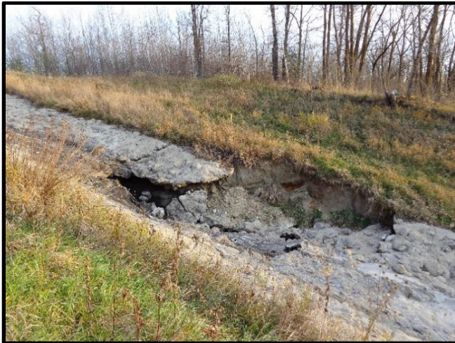
Failure of outlet rock chute due to erosion
