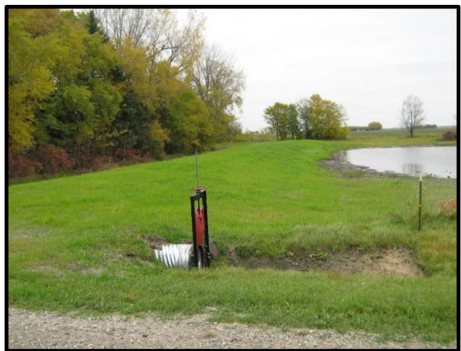
South levee wall and control gate
