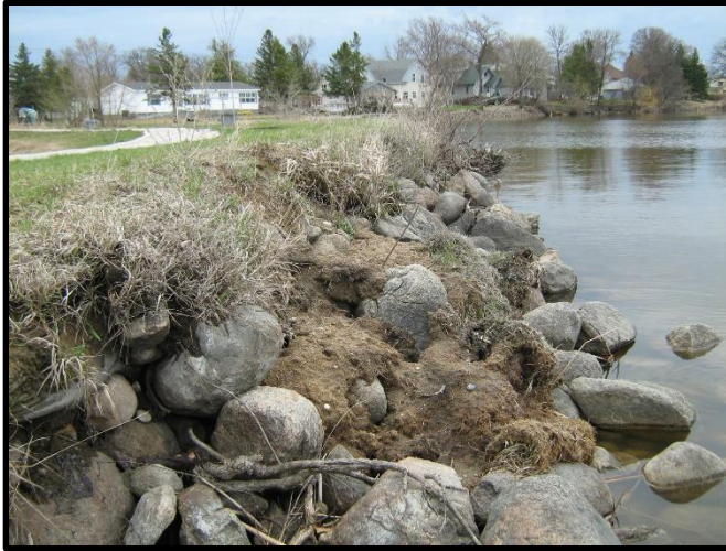
Pre – construction Levee
