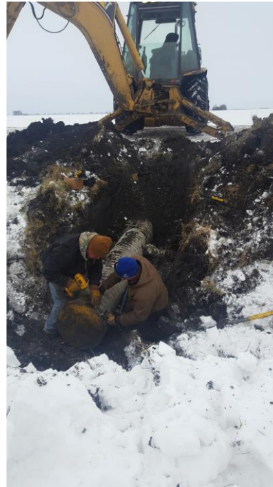
End section of pipe and trap repaired
